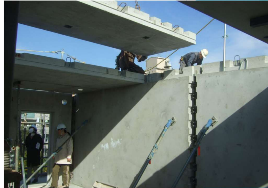
2. Slab panel installation
