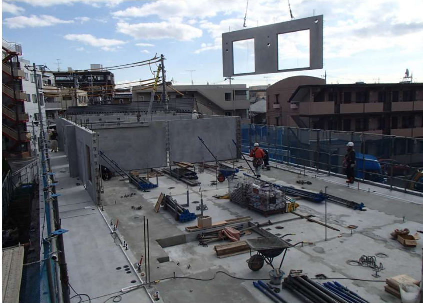
1. Wall panel installation
