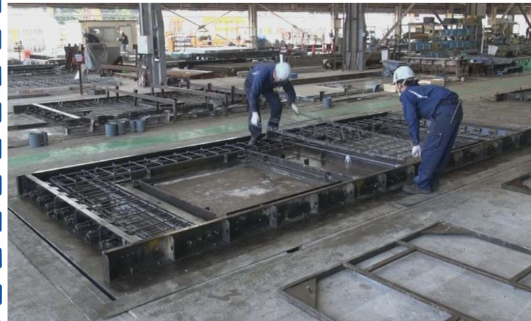
Rebar arrangement works
