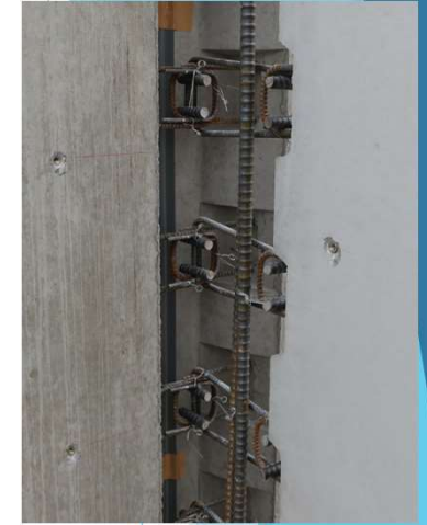
Rebar work of Vertical joints
