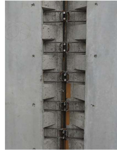
Rebar work of Vertical joints
