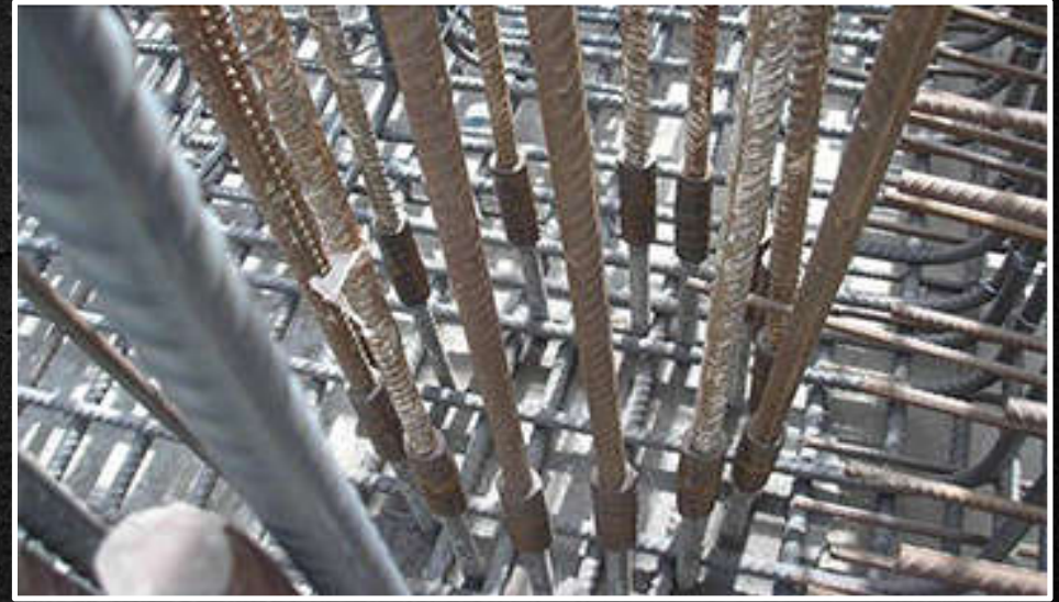
Reinforcement with Mechanical Splicing
