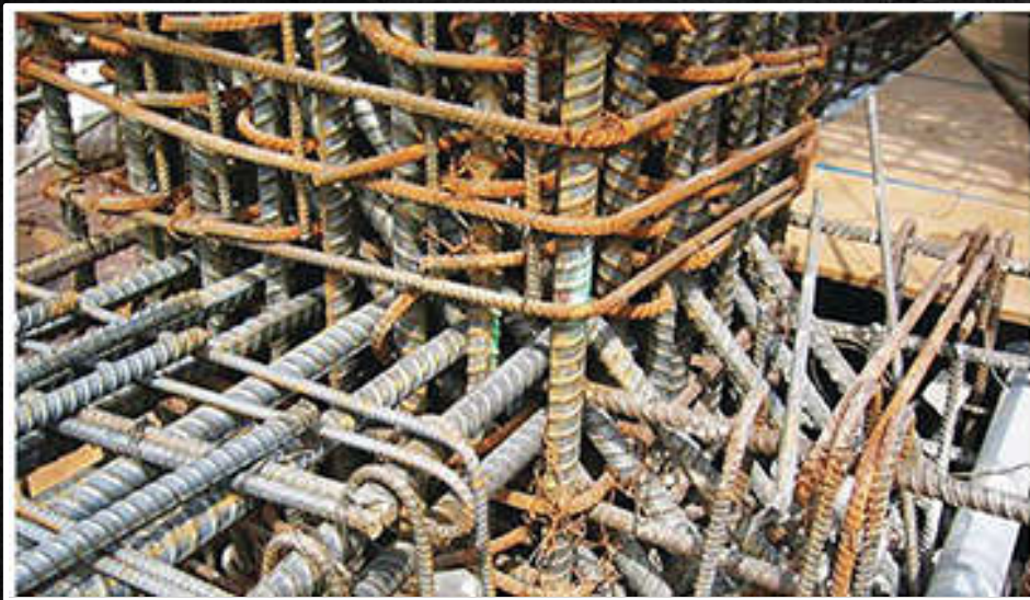
Congestion due to lap splicing
